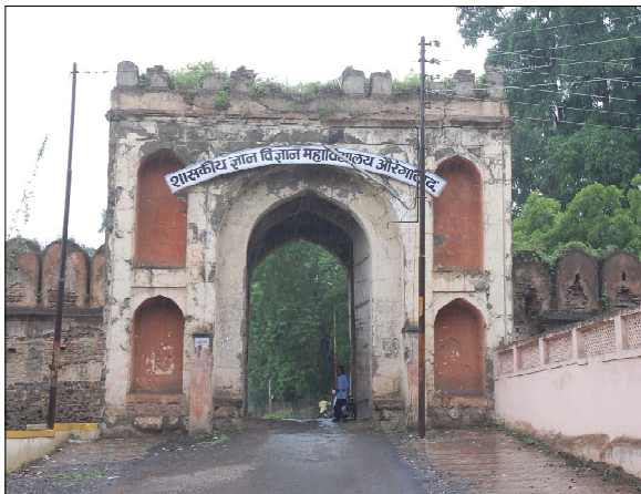
Heritage Buildings Of College : Adil Darwaja
